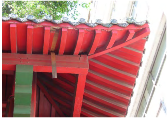
Figure 4.17 Underside of upper roof on the western bay with deteriorated, delaminating plywood soffit.
