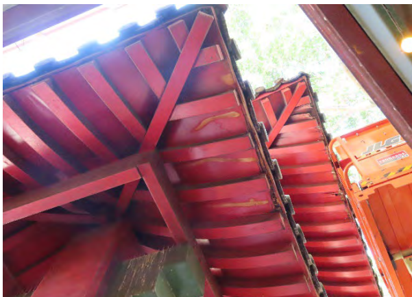
Figure 4.43 Underside of roof timber rafters are in moderate to good condition.
