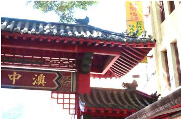
Figure 4.39 Decorative panels including timber lattice C on the western bay of the north elevation.
