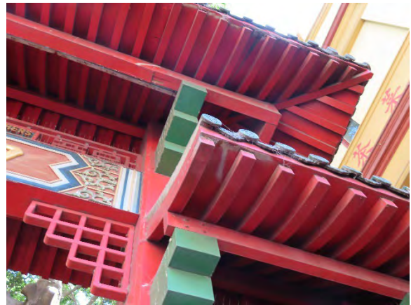
Figure 4.46 View of the exposed roof structure and decorative lattice brace C.
